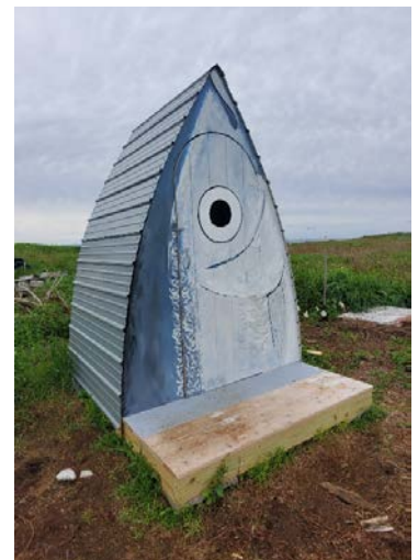
Creature comforts! A new pit toilet was installed this year at Eastern Egg Rock. A microburst destroyed the original one late last season. Photo: Don Lyons
